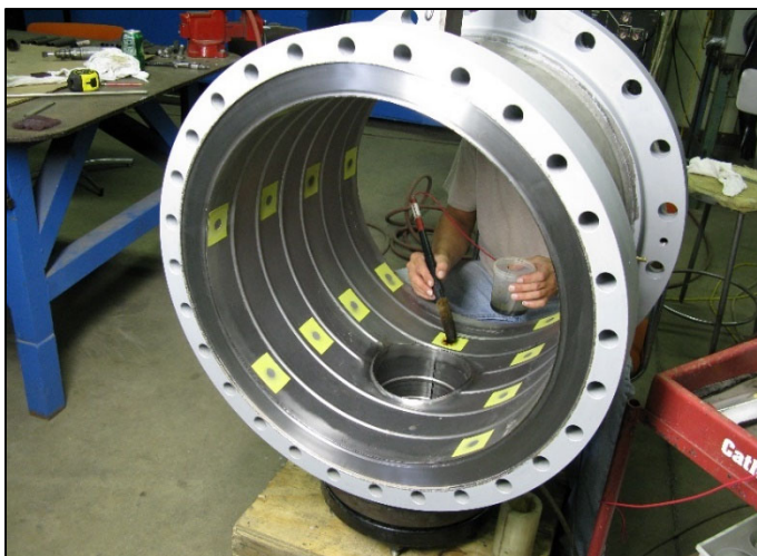
Figure 1 - Platinum spot plating being applied on tantalum lined heat exchanger bonnet.
